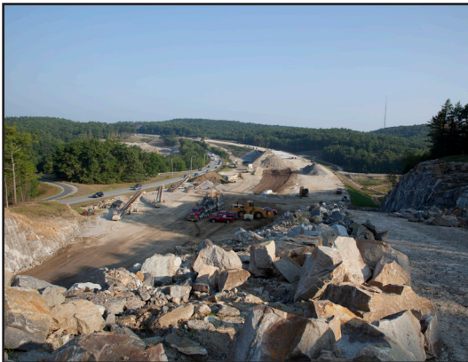
Construction at Exit 3 on I-93
